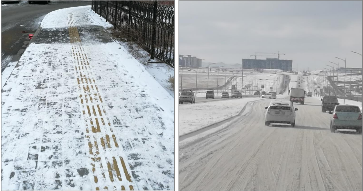
Hazardous tactile paving in a new walkway in Ulaanbaatar.
