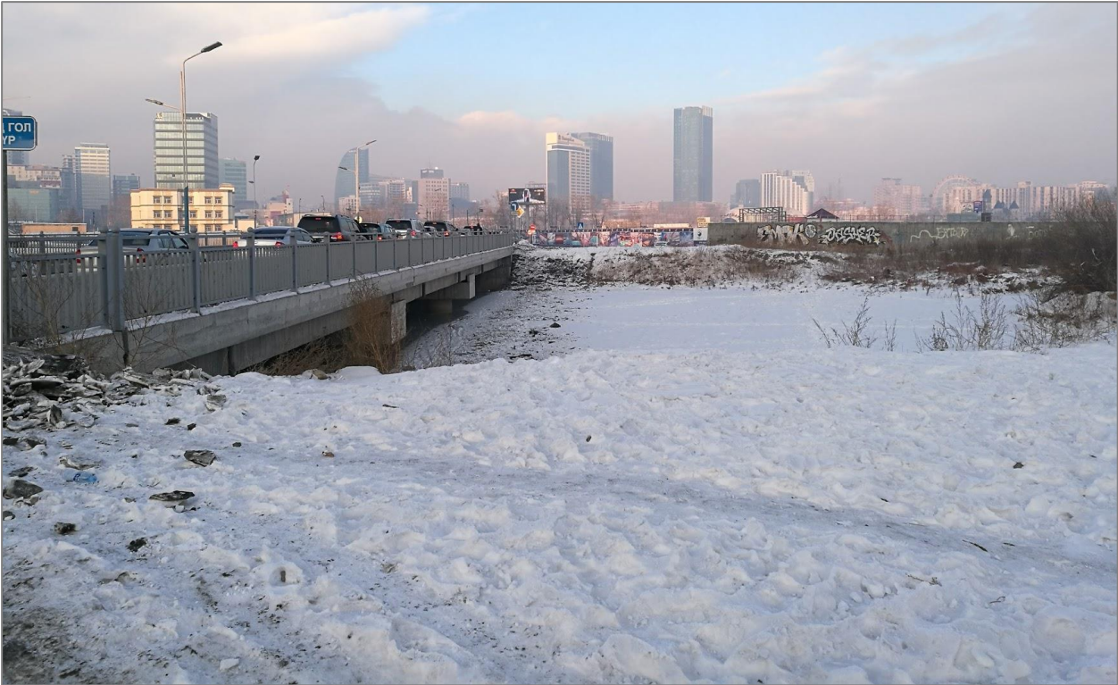
While it would probably be possible to use the existing low bridge to cross this waterway, a BRT-only crossing is preferable.
