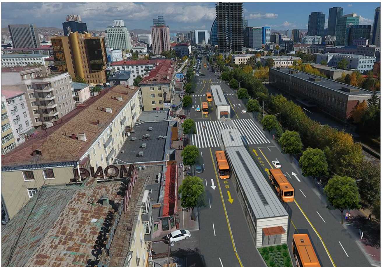
Peace Avenue (station p12 - Baga Toiruu) -- NOTE: the platform location has been changed to either side of the intersection, enabling the pedestrian tunnel to be retained.
